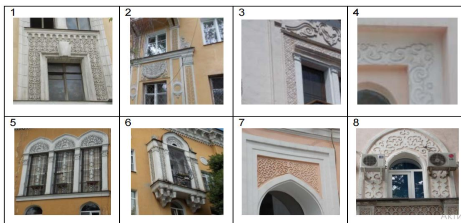
1 – Residential building, Zhibek Zholy Ave.; 2 – Residential building, Zhambyl St.; 3 – Residential building, Tole bi; 4 – Kazpotrebsoyuz Club, Bogenbai Batyr St.; 5, 6 – Residential building, Abylai Khan Ave.; 7 – Kazpotrebsoyuz House, Tole bi St.; 8 – House of Arts, Gogol St.; (Almaty city)
